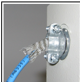
Fig. 6: PANEL EXTERIOR: Both the Ethernet cable and the braided shield must be grounded to the panel enclosure by the cable clamp.
